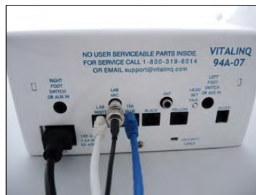
Connection of ethernet, coaxial and power cables to console
